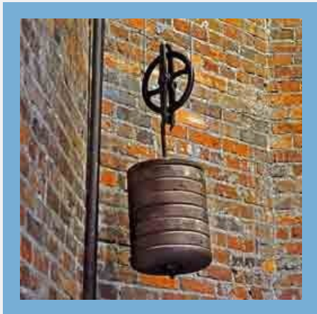
Cast Iron Crane Counterweight
